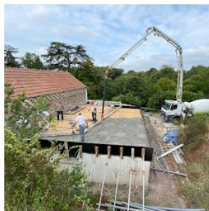
Les Ruchères' worksite
